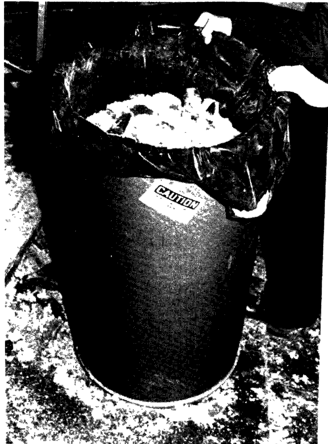
Figure 10. Plastic-lined cardboard container with asbestos waste.
